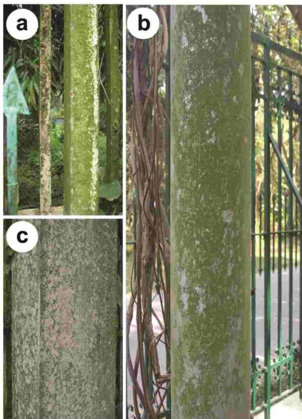
**Figure 1. a – b. Growth of *Apatococcus lobatus* on painted iron surfaces, c. Corrosive activities of the growth of algae on eroded surface of painted iron surfaces**
